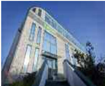
Enerdoor/Finmotor headquarters Milan, Italy
