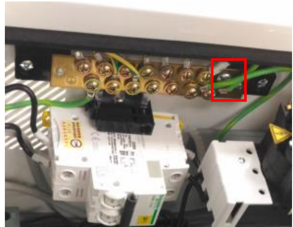
Figure7. 6 Power cable and ground cable installation location
