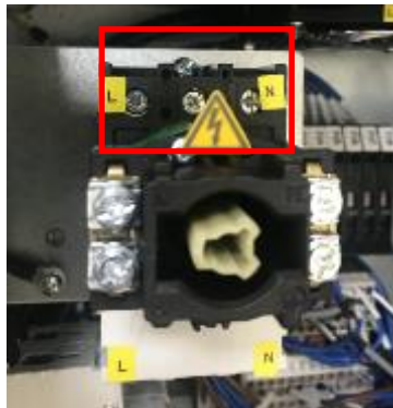
Figure8. 30 Controller power switch primary power check
